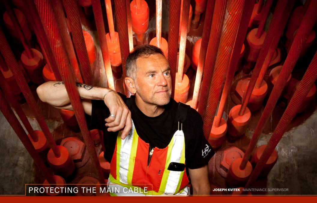
This photo is of the inside of the anchor pier of the MacKay Bridge. It is where the main cable anchors to the concrete. One of the projects on the MacKay in the future will be to install a dehumidification system on the main cable to stop further corrosion. A similar project was completed on the Macdonald Bridge as part of the Big Lift.
